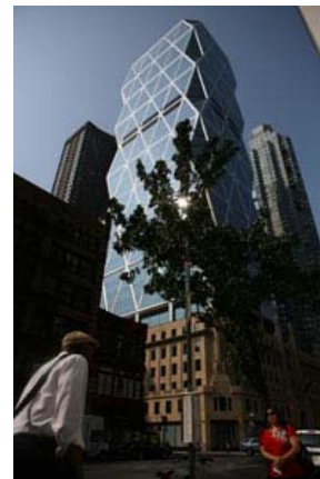
Emmanuel Dunand/ Getty Images The Hearst Tower was the first gold LEED-certified building in New York City. See more green living pictures .
